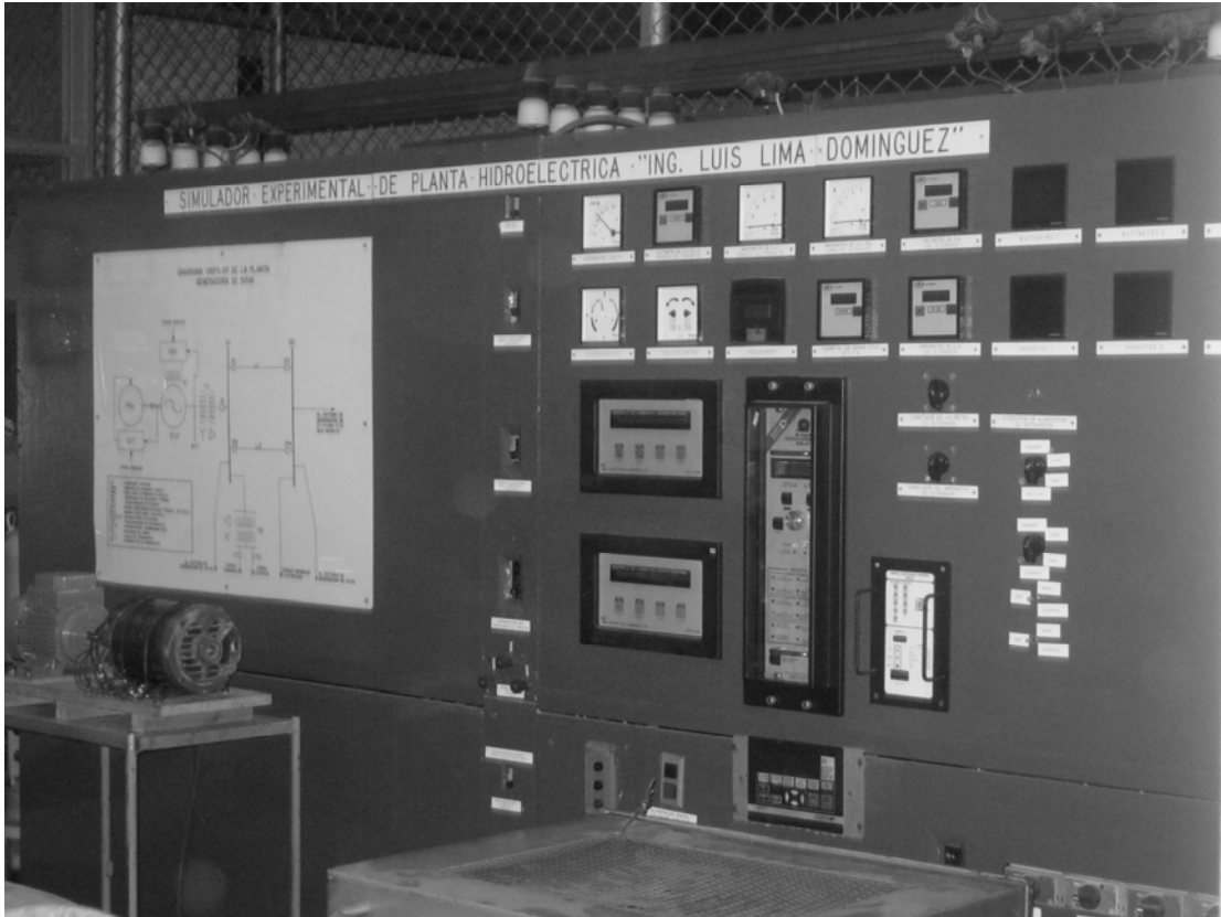
Figura B. 2 Tablero de control del simulador experimental “Ing. Luis Lima Domínguez”
